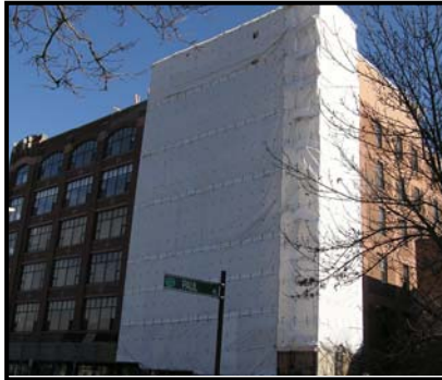
2. Building was staged with winter protection
