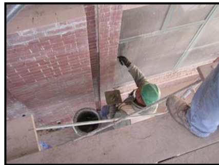
7. Result: Building is successfully restored, with no interruption to users
