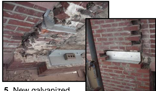
5. New galvanized steel lenticular supports were installed
