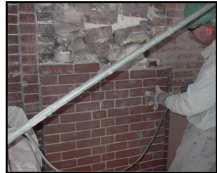
3. Affected areas were demolished
