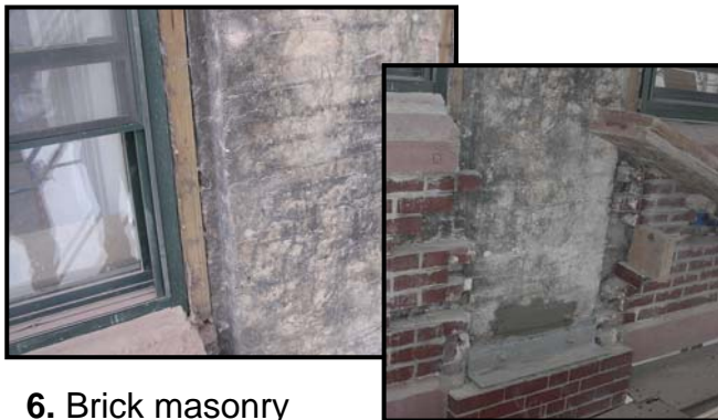
4. Structural repairs were made to building substrate
